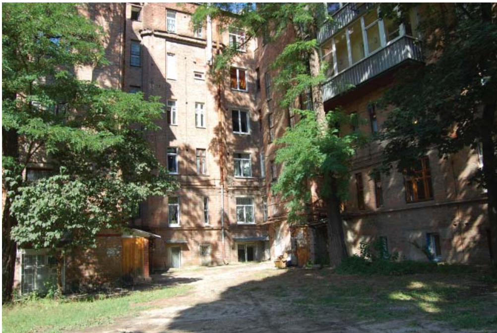
The internal yard of Budynok Slovo. Kharkiv, Ukraine (2008).
